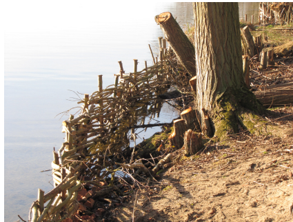
Example of spiling to protect the bank
